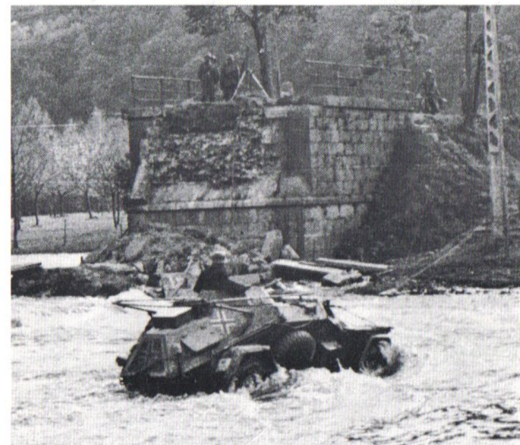
(Below) This Sd.Kfz. 223 radio vehicle fords a stream next to a destroyed bridge during the French campaign of 1940. The large frame antenna has been folded down to provide the vehicle's gunner with a clear field of fire if the necessity arises. The vehicle also carried a long whip antenna which was stowed on the side of the vehicle and could be erected whenever desired. It was used for transmission, while the frame antenna was used to receive signals.
