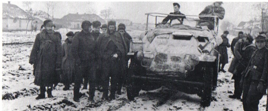
(Below) A scene from Russia, 1943. Escorting prisoners to the rear, this Sd.Kfz. 261 radio car sports an MG 42 as its protective armament. This vehicle is from the signals regiment of the 24th Panzer Division . The Sd.Kfz. 260 and 261 differed from the Sd.Kfz. 223 in that they had no turrets, while the 223 did.
