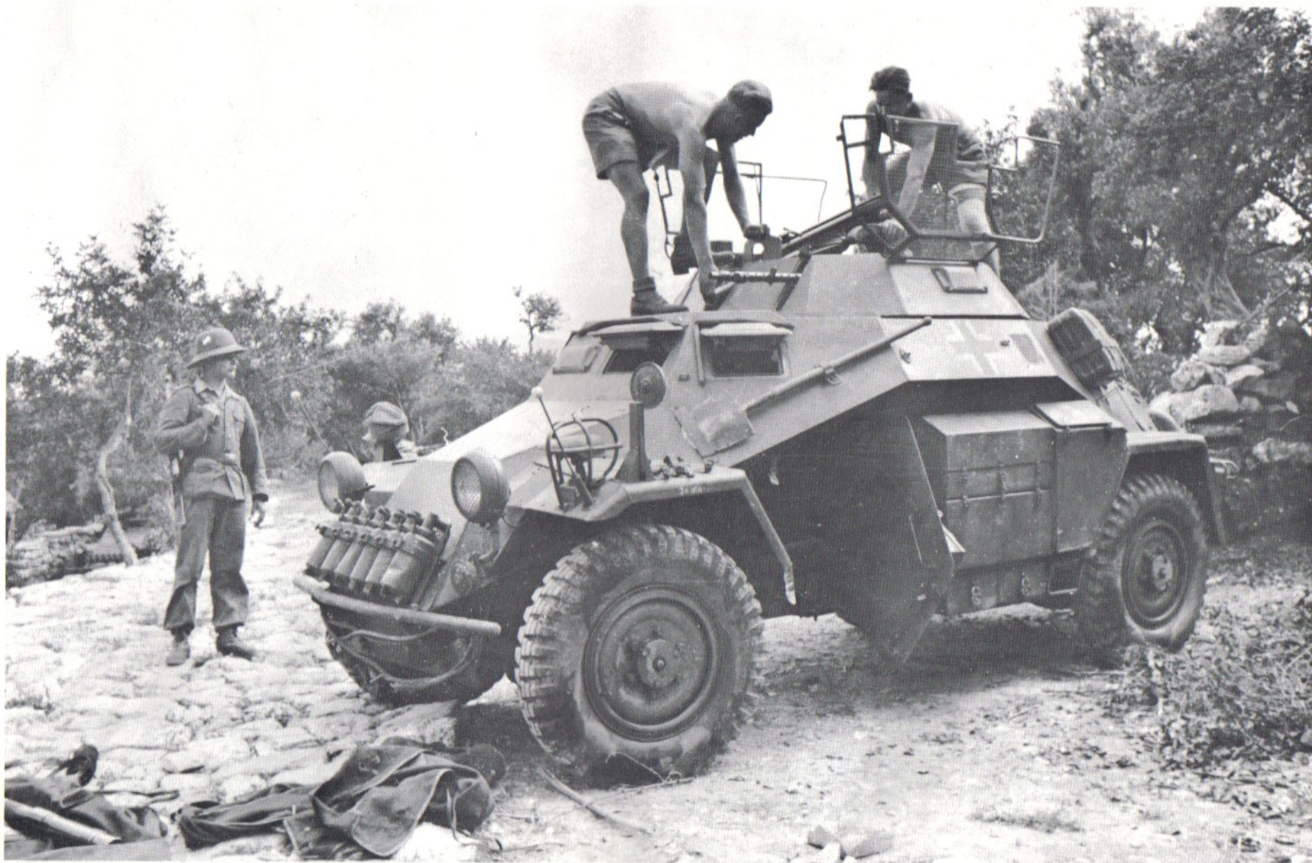
Here, the crew of an Sd.Kfz. 222 is in the process of removing the breech and visible on the tarpaulin on the ground at the left of the photo is the barrel recoil mechanism of their 20mm main armament, in order to clean it.
